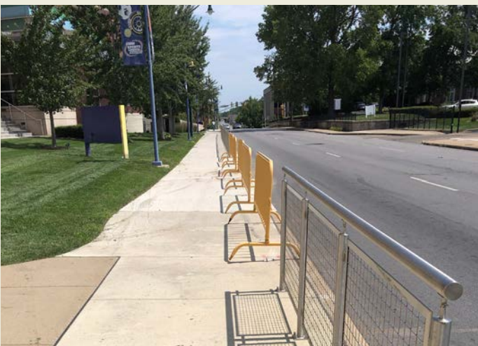
Pedestrian-scaled railings offer protection for pedestrians from stumbling into three lanes of one-way traffic along the north side of W. 30th St. outside the Children's Museum of Indianapolis. The railings were installed as part of the Red Line bus rapid transit infrastructure enhancements. Located east of intersection with N. Illinois St. (Crash Zone 9).
