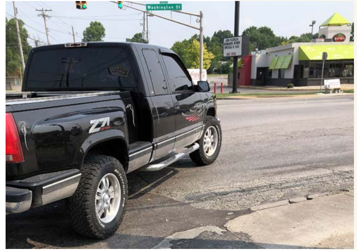
A motorist turns right onto W. Washington St. from S. Lynhurst Dr. Discontinuous sidewalk is present at each of the intersection's four corners; however, layering of asphalt over time has rendered some curbs useless, leaving pedestrians vulnerable to being hit by turning vehicles cutting the corner. Crosswalks are non-existent.
