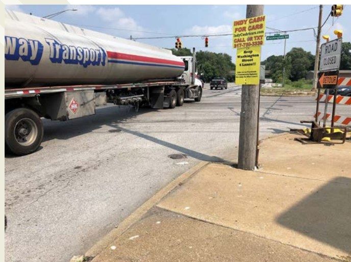
Viewed from the southeast corner of the intersection of W. Washington St. and Holt Rd., a semitruck runs a red light. Meanwhile, ADA-compliant curb ramps and high-visibility crosswalks are absent from the intersection. Furthermore, utility poles and temporary construction signage present obstructions for pedestrians. A sign on the utility pole reads "Keep Washington Street 4 Lanes!!!" in reference to IndyGo's planned Blue Line bus rapid transit project, which would introduce even basic pedestrian infrastructure to the corridor.
