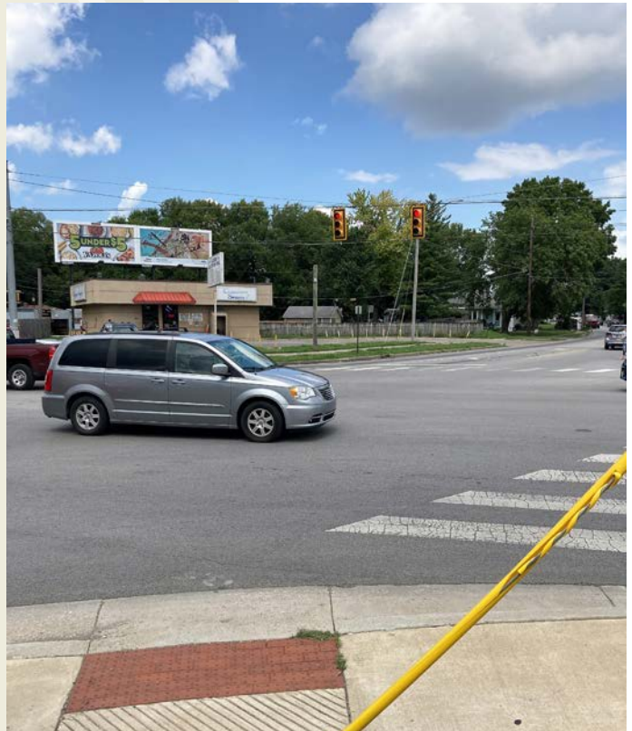
At the time of the walk audit, the busy intersection of W. 10th St. and N. Tibbs Ave. included high-visibility crosswalks in good condition, clear and unobstructed sidewalks, and ADA curb ramps. However, the detectable warning system was improperly installed and is misaligned with the diagonal crosswalks, posing danger to persons with no or low vision.
