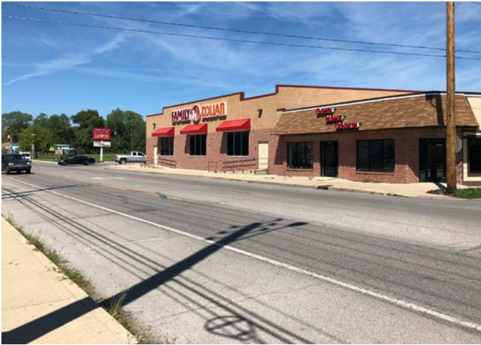
Community assets, like this Family Dollar on the east side of the intersection of Dr. Martin Luther King Jr. St. and W. 26th St., need to be safe and accessible for people walking from the west side of the street. The closest crosswalks are about 350' to the northwest and 600' to the southeast (Crash Zone 8).
