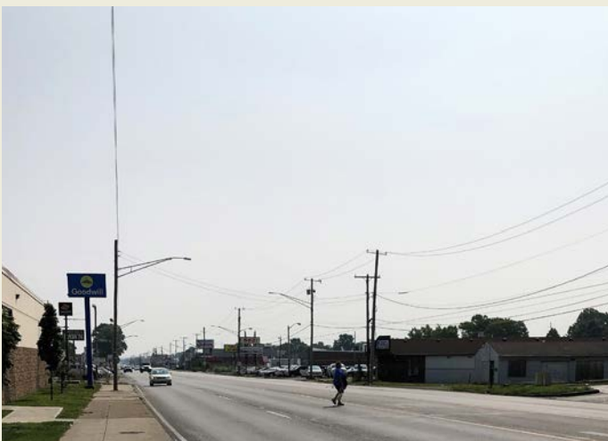
A lone pedestrian crosses five lanes of W. Washington St. Few blocks throughout the corridor include newer, ADA-compliant sidewalks, curb ramps, and crosswalks; however, a lack of stoplights or other traffic controls create few opportunities for pedestrians to cross safely—oftentimes up to a ½-mile from the nearest signalized intersection.
