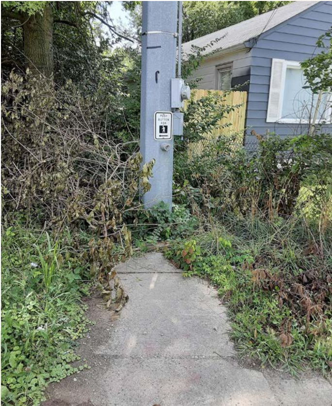
A pedestrian push button is tucked away from the mainline sidewalk and surrounded by overgrown brush at the southwest corner of the intersection of W. Michigan St. and Holt Rd. This is also one of only two pedestrian crossings at the intersection.
