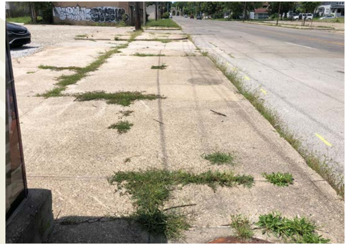
In the foreground, weeds and grass begin to cause an impediment to this section of sidewalk on the south side of W. 34th St. In the background, pre-ADA curb cuts for motor vehicles do not accommodate pedestrians in wheelchairs or other mobility devices. Intersection of N. Illinois St. and W. 34th St. (Crash Zone 9).
