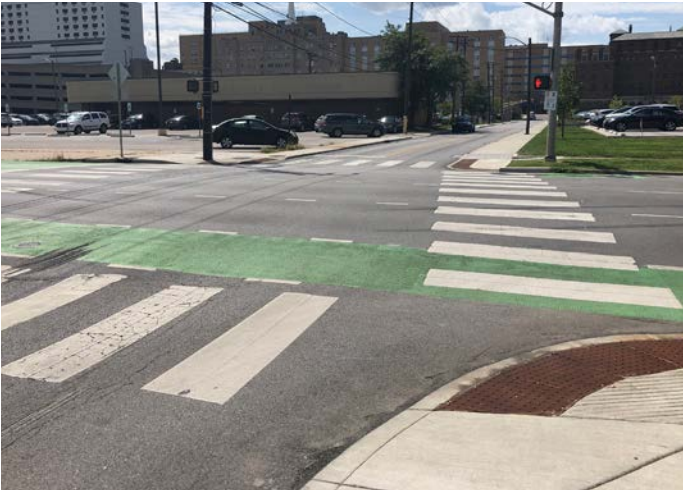
Freshly painted bike lanes and crosswalks as part of the Red Line bus rapid transit infrastructure enhancements. Intersection of W. 18th St. and N. Illinois St. (Crash Zone 9).
