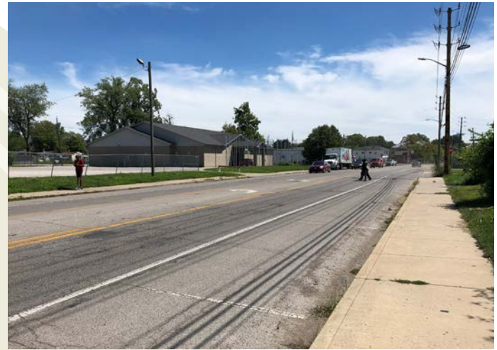
Pedestrians crossing at the intersection of Dr. Martin Luther King Jr. St. and W. 26th St. There are minimal opportunities for pedestrians to safely cross the busy street (Crash Zone 8).
