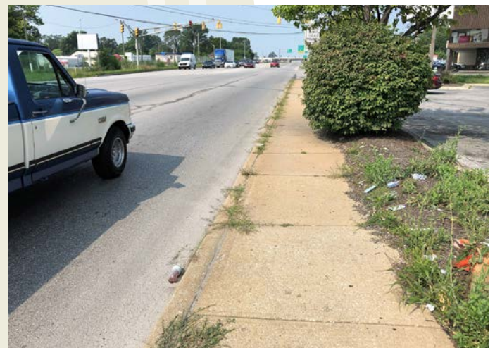
Overgrown shrubs block a portion of sidewalk on W. Washington St. near its intersection with Waldemere Ave. and W. Morris St., forcing pedestrians to walk uncomfortably close to traffic typically traveling 40 miles per hour or higher. Weeds and litter contribute further to an inhospitable walking environment.
