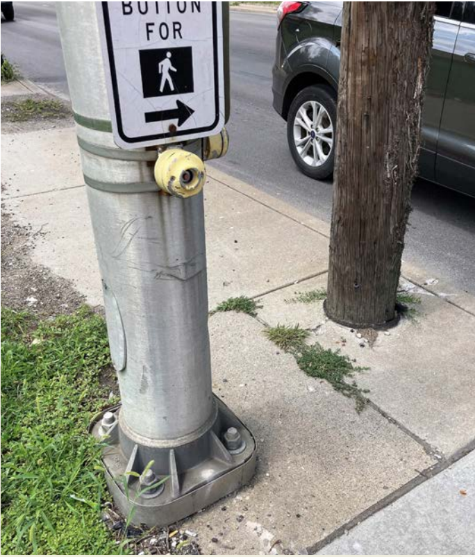
A traffic signal post (left) and utility pole (right) on the southwest corner of the intersection of W. 10th St. and N. Concord St. The placement of these poles on the sidewalk creates an impassable barrier to persons using mobility devices. The splintered wood of the utility pole facing 10th St. indicates that there may be a history of excessive speeds or reckless driving among passing motorists.
