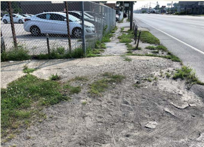
A blending of discontinuous sidewalk segments, asphalt surface parking lots, and gravel shoulders are a common sight throughout the corridor. This photo was captured at the northeast corner of W. Washington Street's intersection with S. Worth Ave. looking east.
