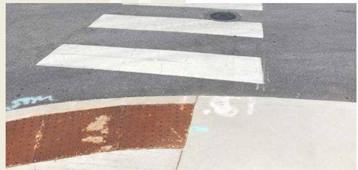
Freshly painted crosswalks and ADA-compliant curb ramps were observed along the Meridian St. corridor as part of the Red Line bus rapid transit infrastructure enhancements. Intersection of N. Meridian St. and E. 37th St. (Crash Zone 4).
