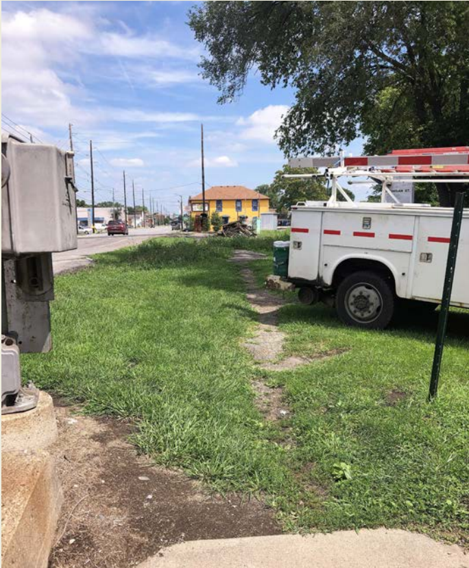
A dirt path is visible looking east along the south side of W. Michigan St. between N. Warman Ave. and railroad tracks provides evidence of a gap in the sidewalk network that should be filled. At the time of this report's publication, pedestrian enhancements were underway at this intersection as part of the B&O Trail extension.
