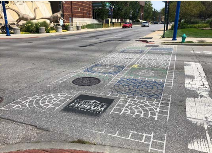
Another weathered duratherm crosswalk outside the Children's Museum of Indianapolis. Intersection of N. Illinois St. and W. 30th St. (Crash Zone 9).
